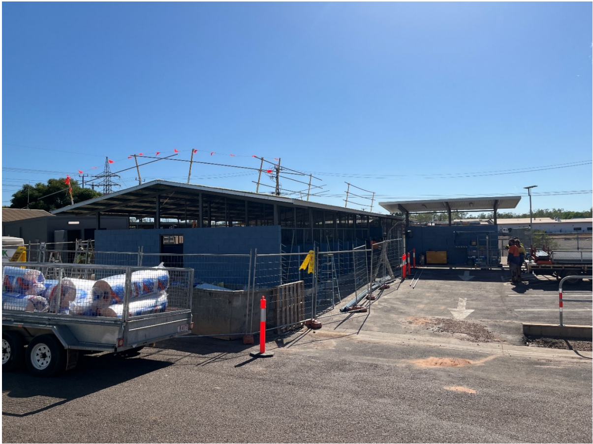
Figure 1: Construction of Animal Management Facility, 27 August 2026
