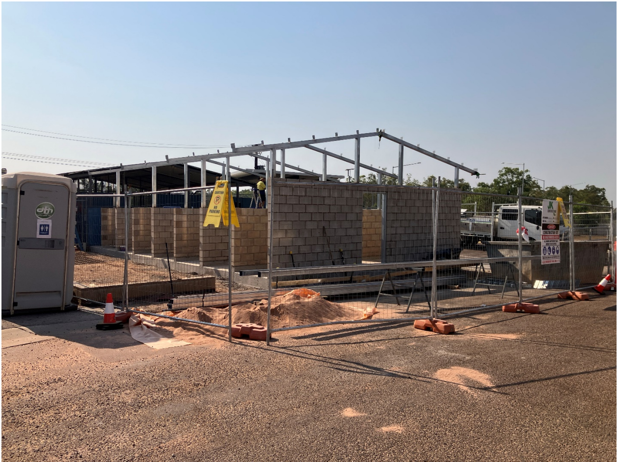
Figure 1: Construction of Animal Management Facility, 30 July 2026
