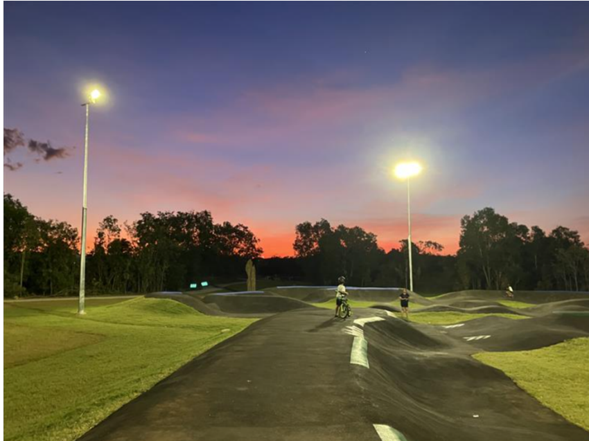
Figure 8: Pump Track Lighting
