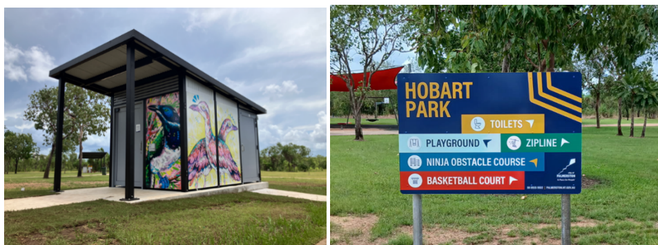
Figure 1: Completed Hobart Park Toilet and Signage
