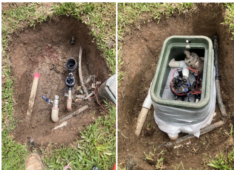
Figure 4: Irrigation upgrade works at Joan Fejo Park, Rosebery
