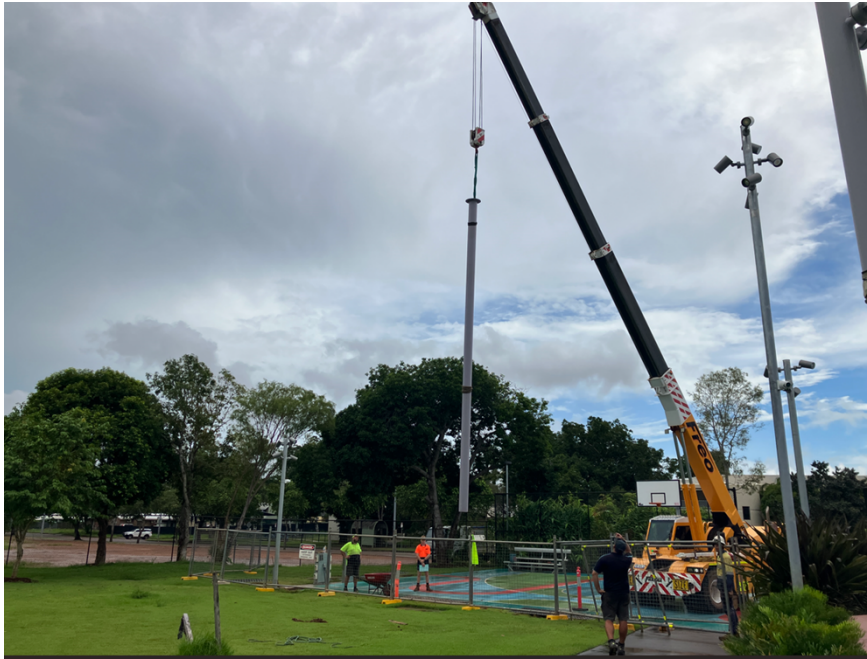
Figure 6: SWELL Basketball shade installation
