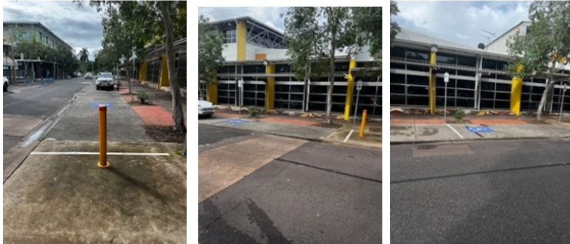
New Parking Bays at Recreation Centre
