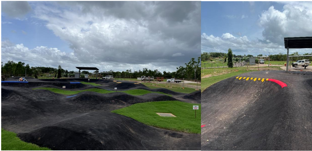
Figure 1: Pump track construction - 18 February 2026
