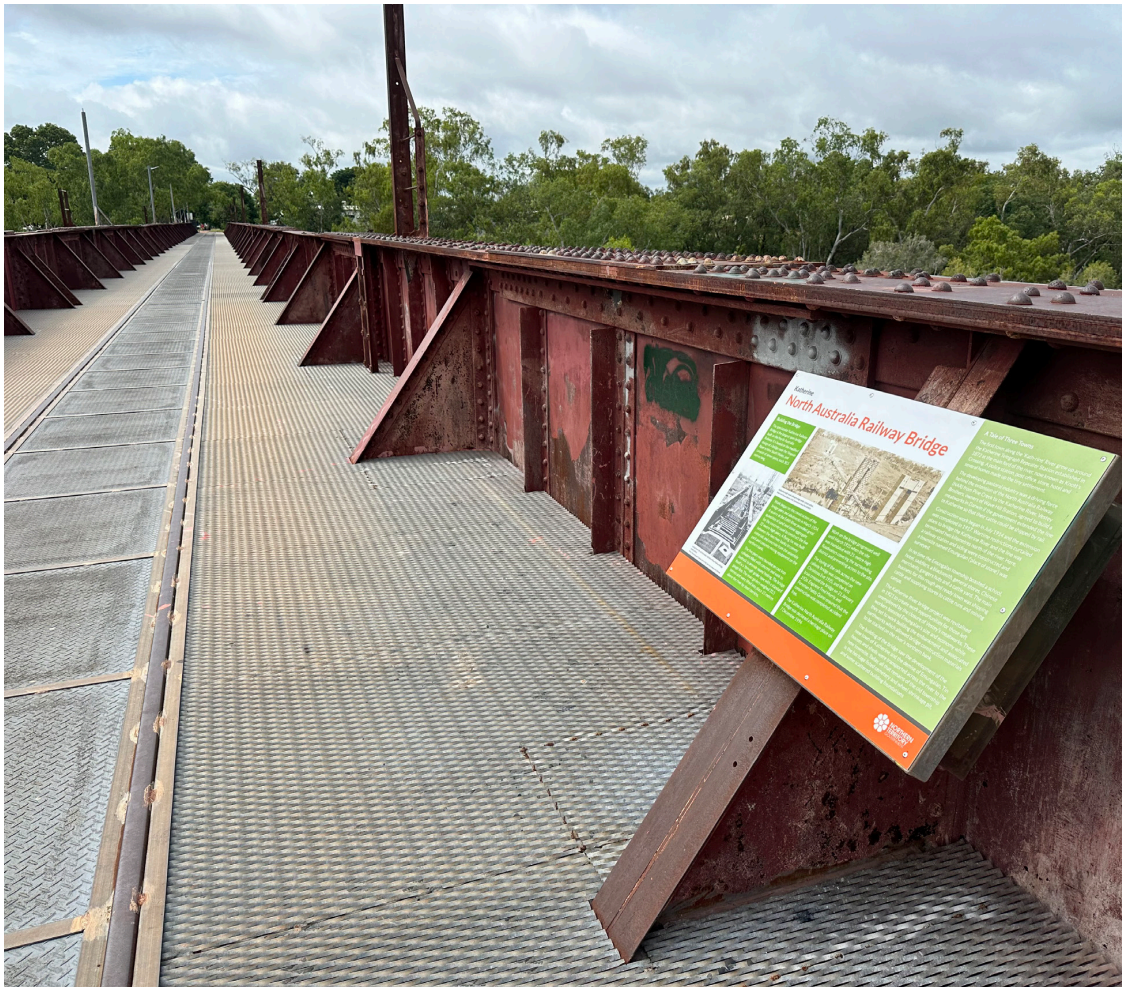
Katherine River Railway Bridge – Updated signage 2024-25
