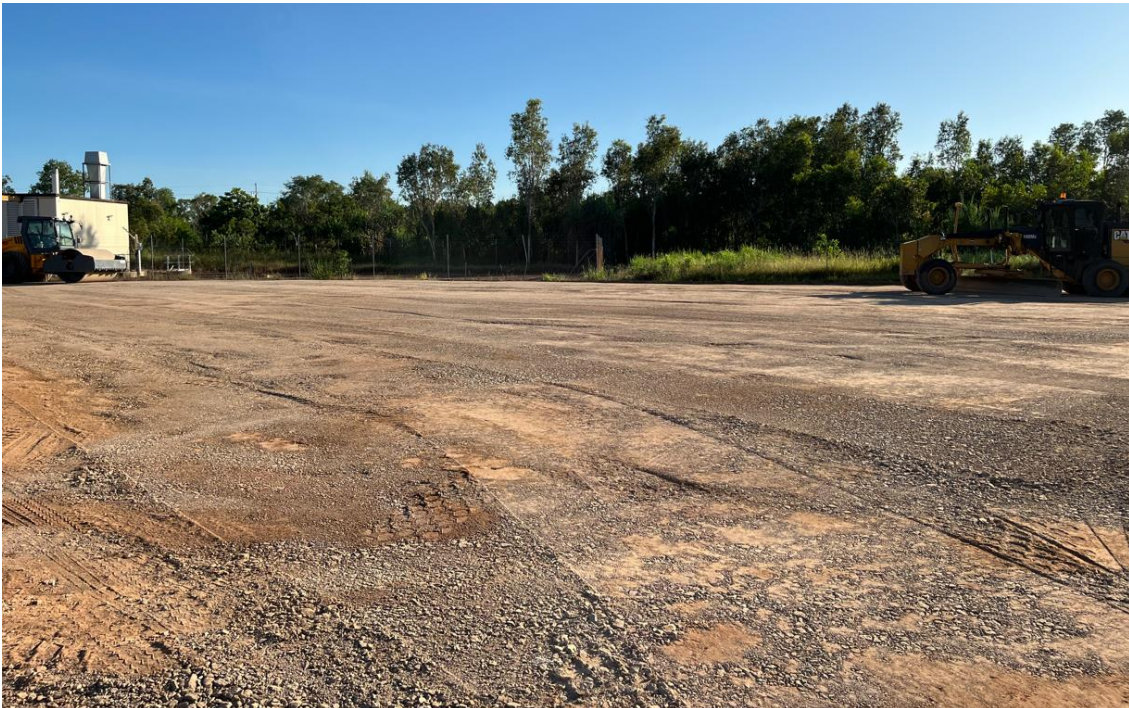
Subgrade Preparation – 5 March 2025
