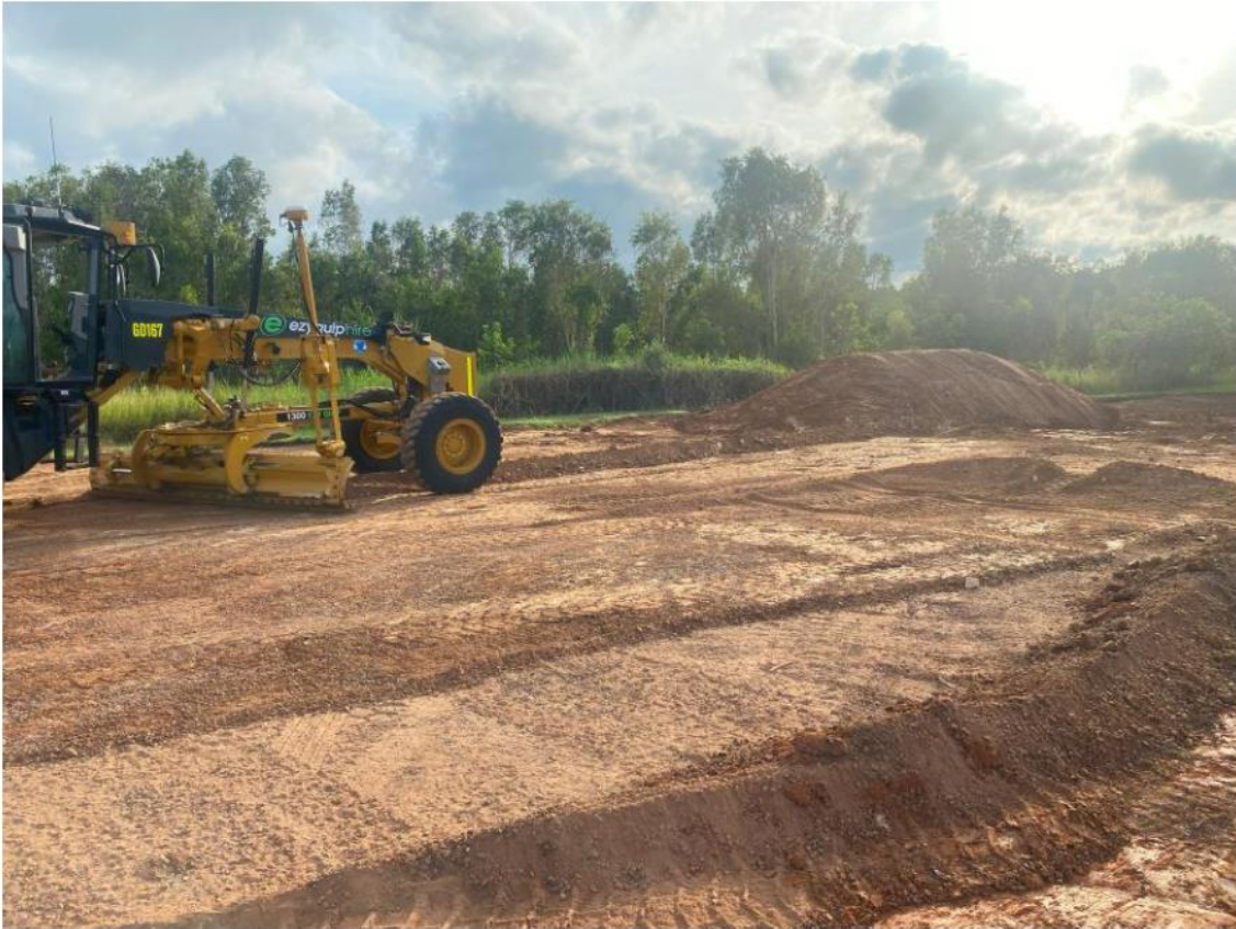
Grader levelling – 24/01/2025
