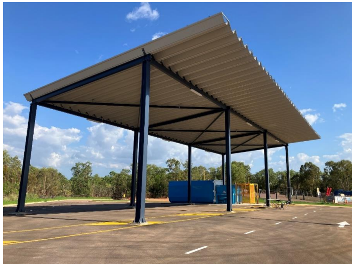
Figure1: 20 October 2025 – Construction Complete
