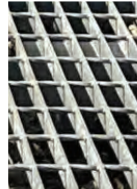
CREEK CROSSING OR AREAS OF INUNDATION - STEEL GRATE DECKING
