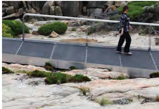
METAL DECK STRUCTURE IN AREAS OF INUNDATION
