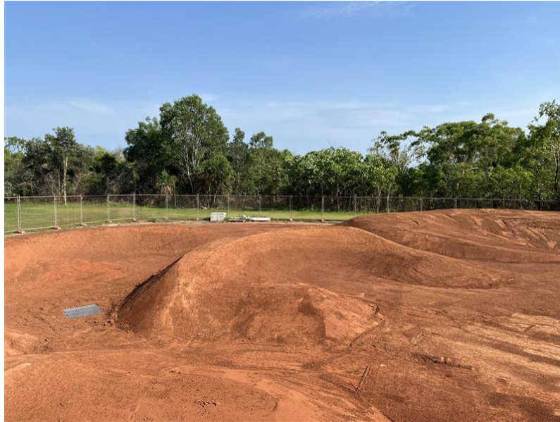
Figure 2: Pump track construction - 5 November 2025
