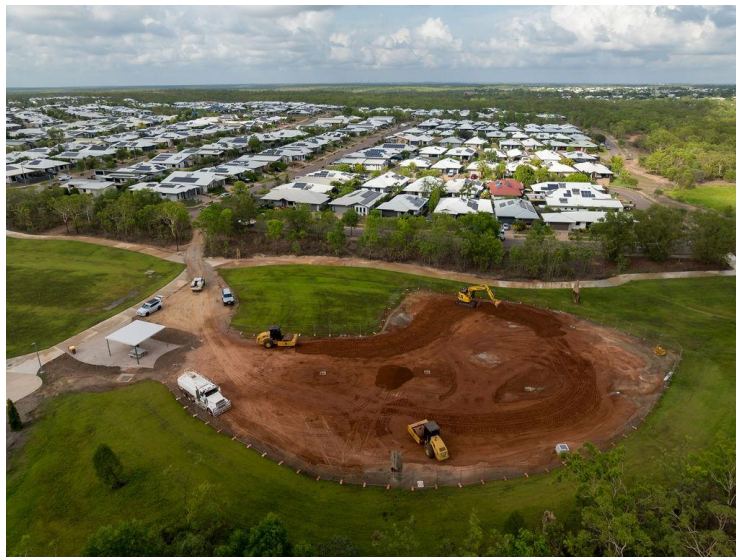
Figure 1: Pump track Construction 8 October 2025
