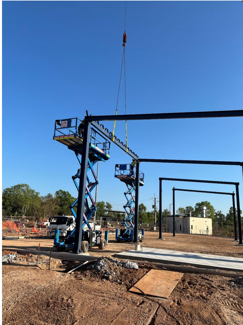
03 September 2025 – Shelter Roof Beam Installation
