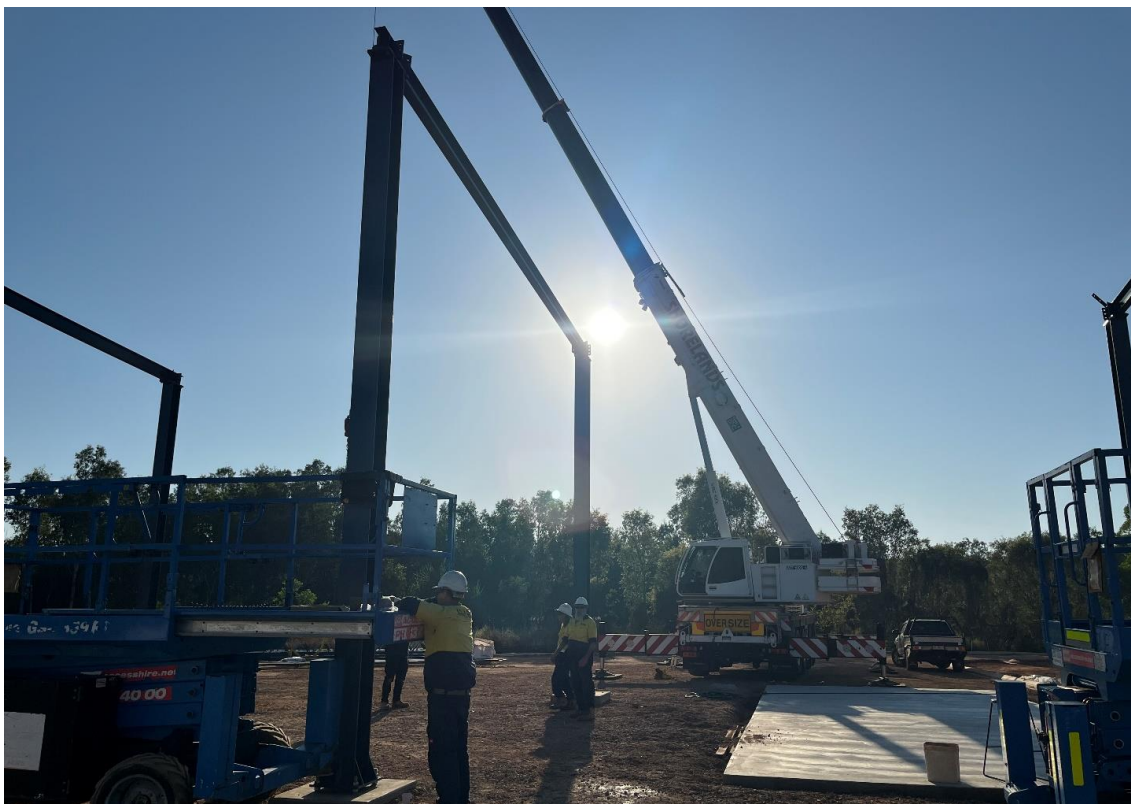
03 September 2025 – Shelter Roof Beam Installation
