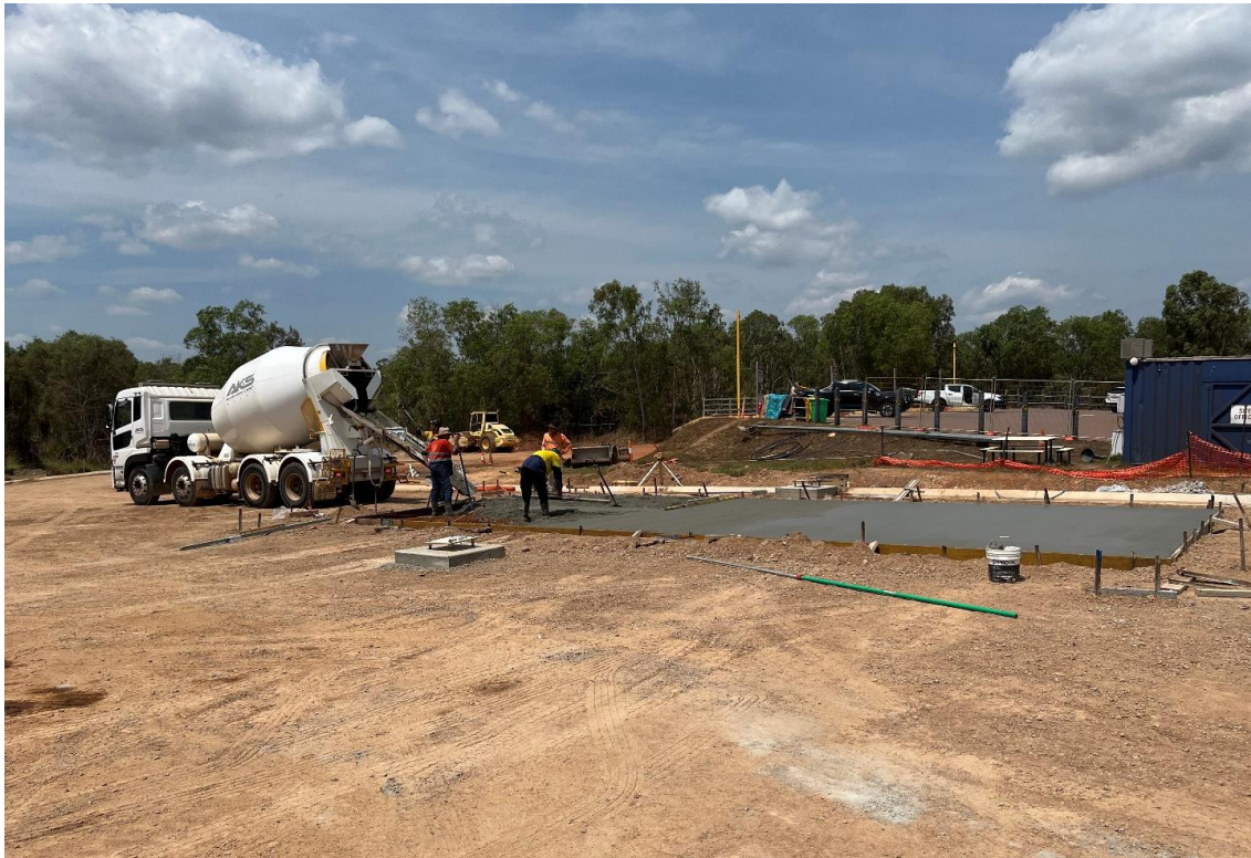
29 August 2025 – Cardboard Compactor Slab installation
