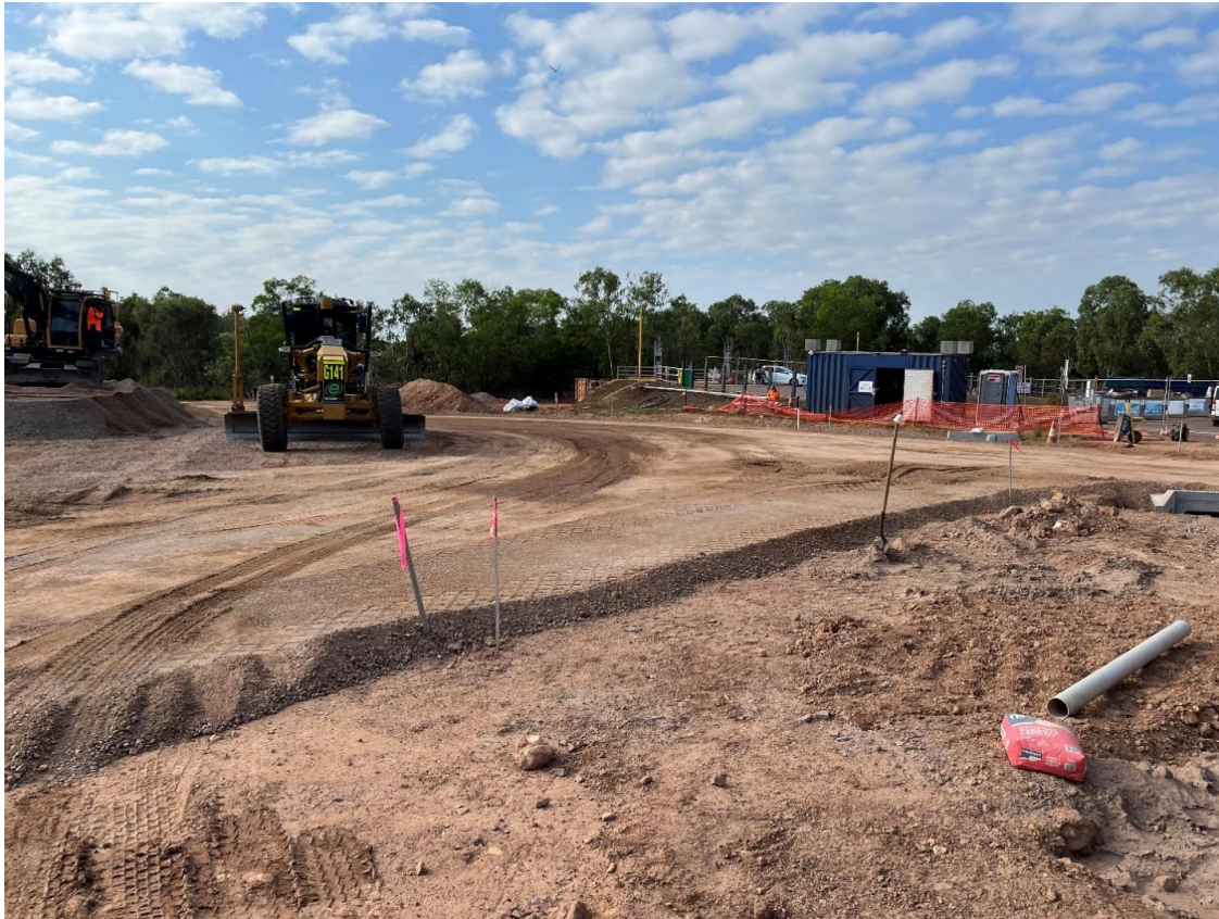
Subbase material being placed
