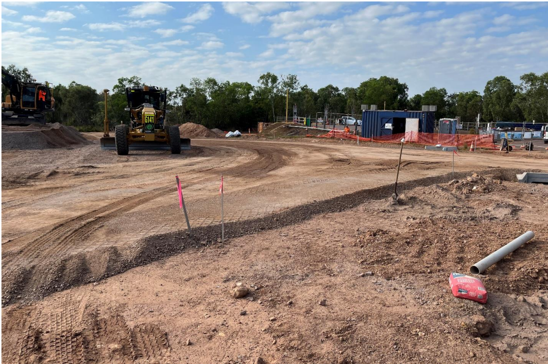
30 July 2025 – Subbase placement and compaction
