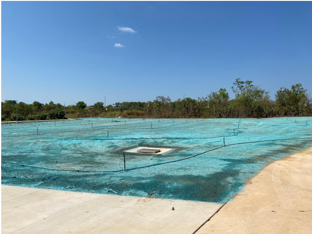
Stage 2 Civil works complete – multi-sports court area hydroseeding
