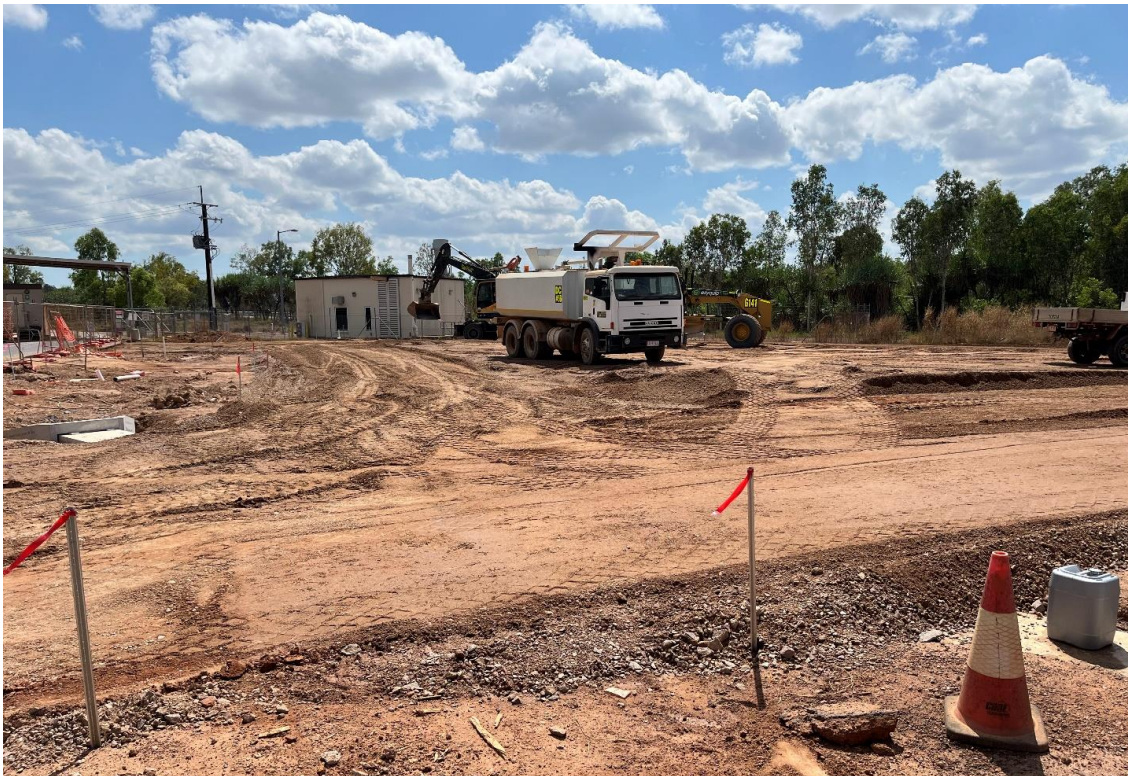
31 July 2025 – Subbase placement and compaction
