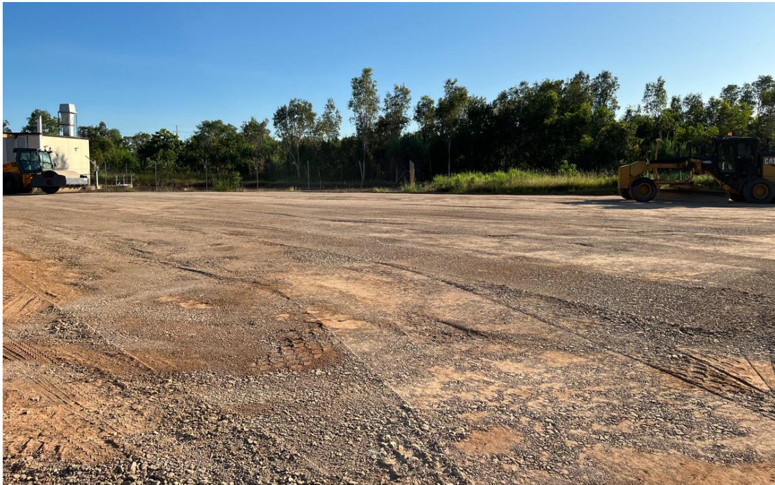
Subgrade Preparation – 5 March 2025
