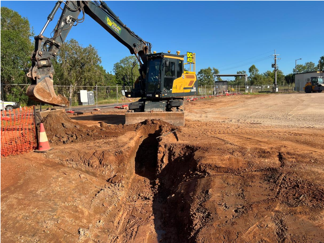
Stormwater Culvert Trenching – 5 th March 2025
