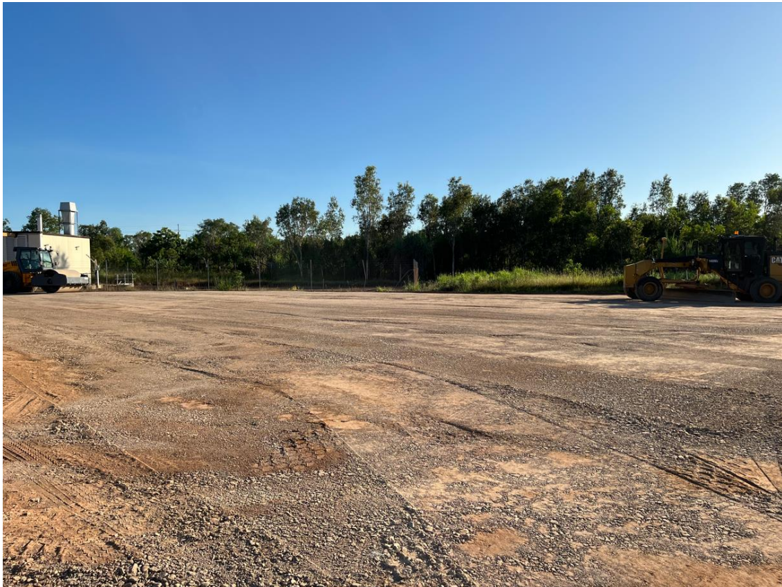
Subgrade Preparation – 5 th March 2025
