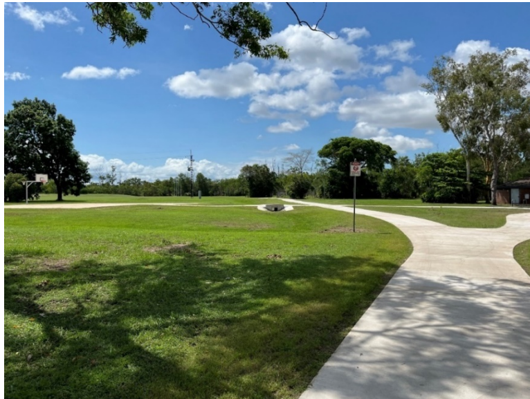
New Pathway – Marlow Lagoon Basketball Court
