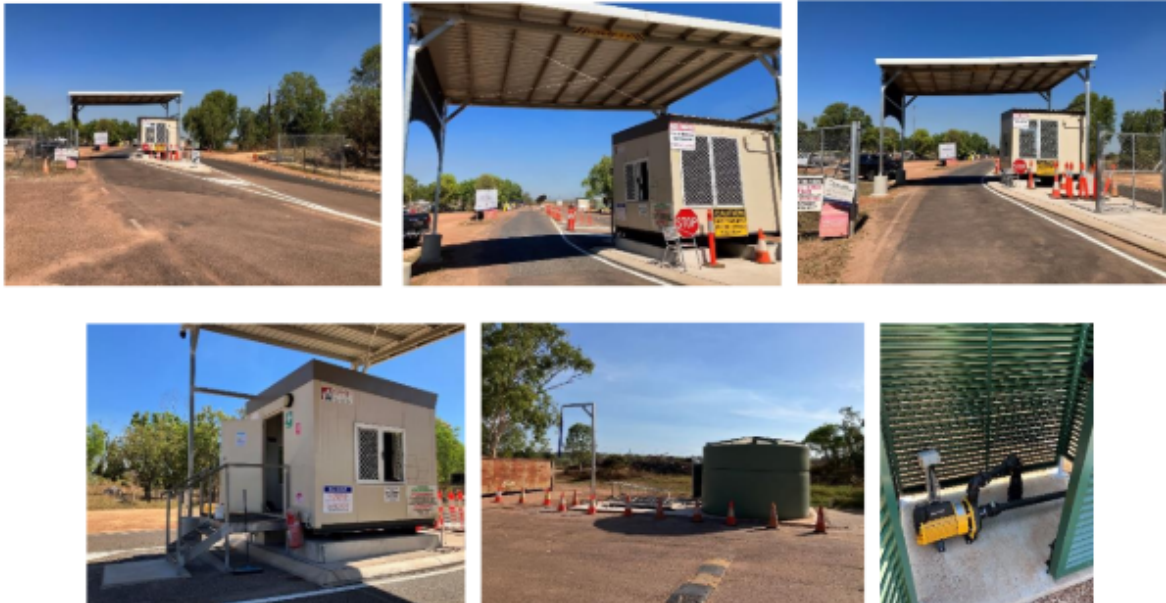
Archer Waste Management Facility
