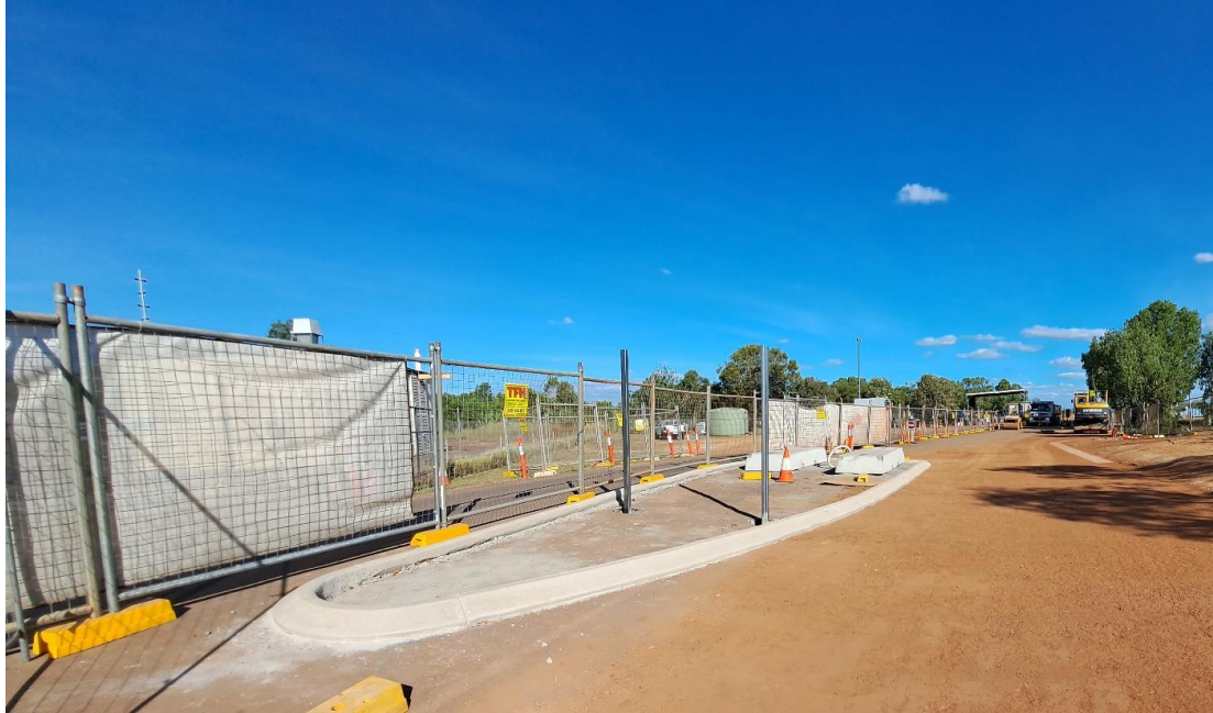
Archer Gatehouse Relocation Siteworks
