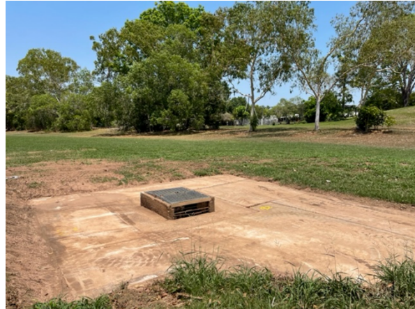
After: Moulden Drain pit 92 and apron
