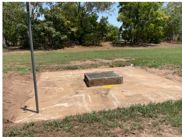
After: Moulden Drain pit 93 and apron
