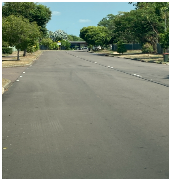
Essington Avenue recently resealed
