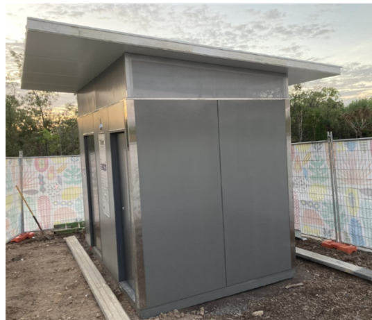
Figure 2 - Dog Park Exeloo Installation – photo 08/06/23
