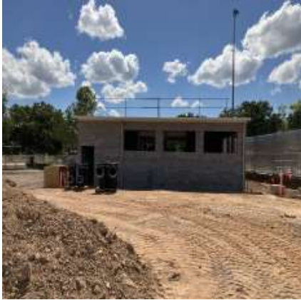
Plant Room structure complete 06/06/23
