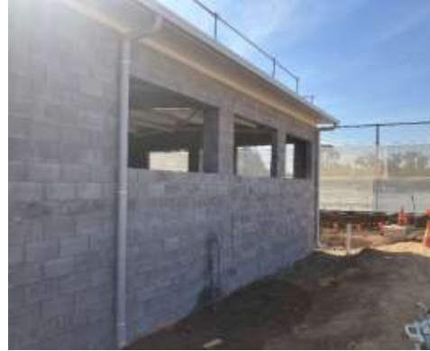
Plant room structure and roof/downpipes 06/06/23
