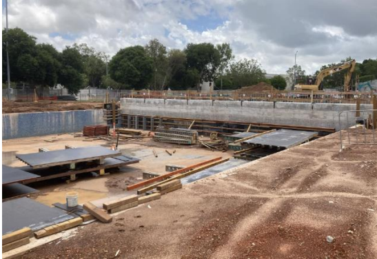
Pool Construction Progress 09/03/2023
