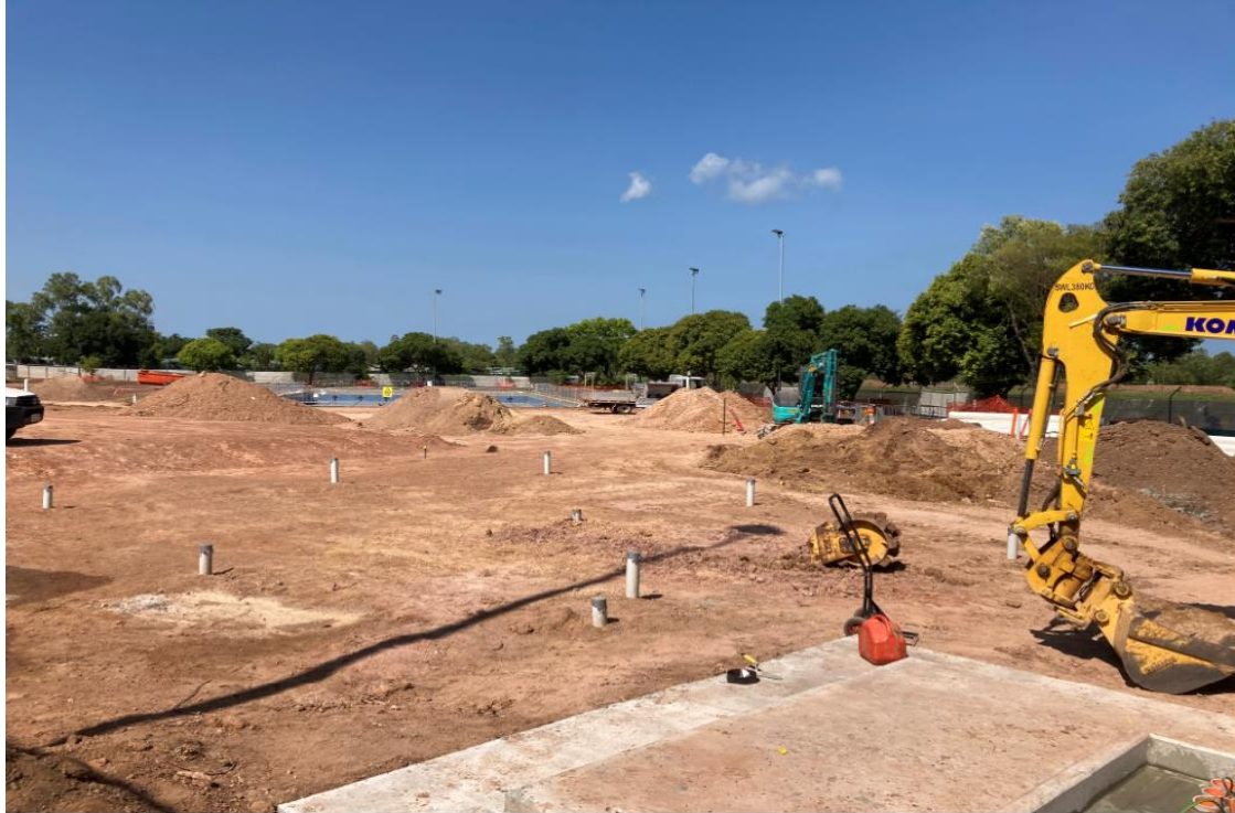
Earth Works and Underground Services
