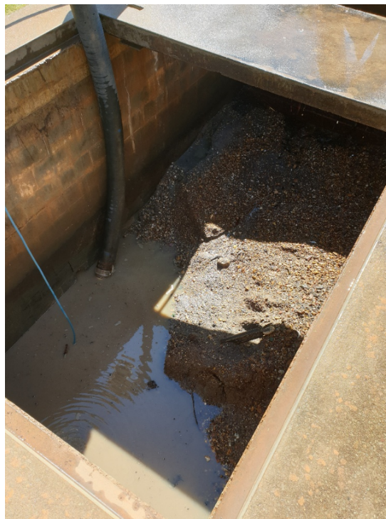
Image 6: Gross pollution trap, Sanctuary Lakes, Gunn stormwater works
