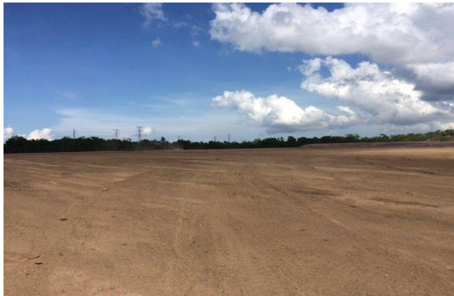
Image 1: Archer landfill rehabilitation stage 1 – completed revegetation layer
