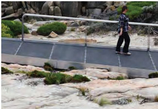
METAL DECK STRUCTURE IN AREAS OF INUNDATION
